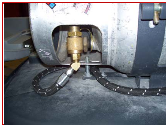
New Hose Routing with More Clearance
