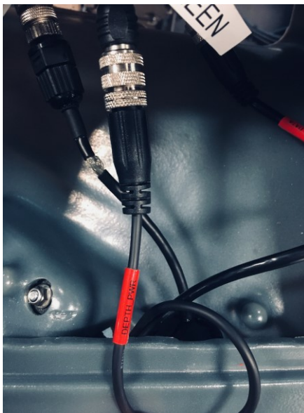
Figure 31: 3D Depth Sensor Power Cable
